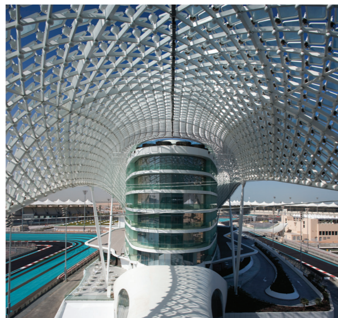
Above: The LED canopy. Opposite page top: Outdoor dining at the Yas Viceroy Abu Dhabi.
